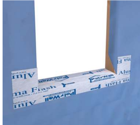
STEP 7 Cut the Aluma Flash™ at the corners of the rough opening so that the Aluma Flash™ may be folded onto the WRB surface.
